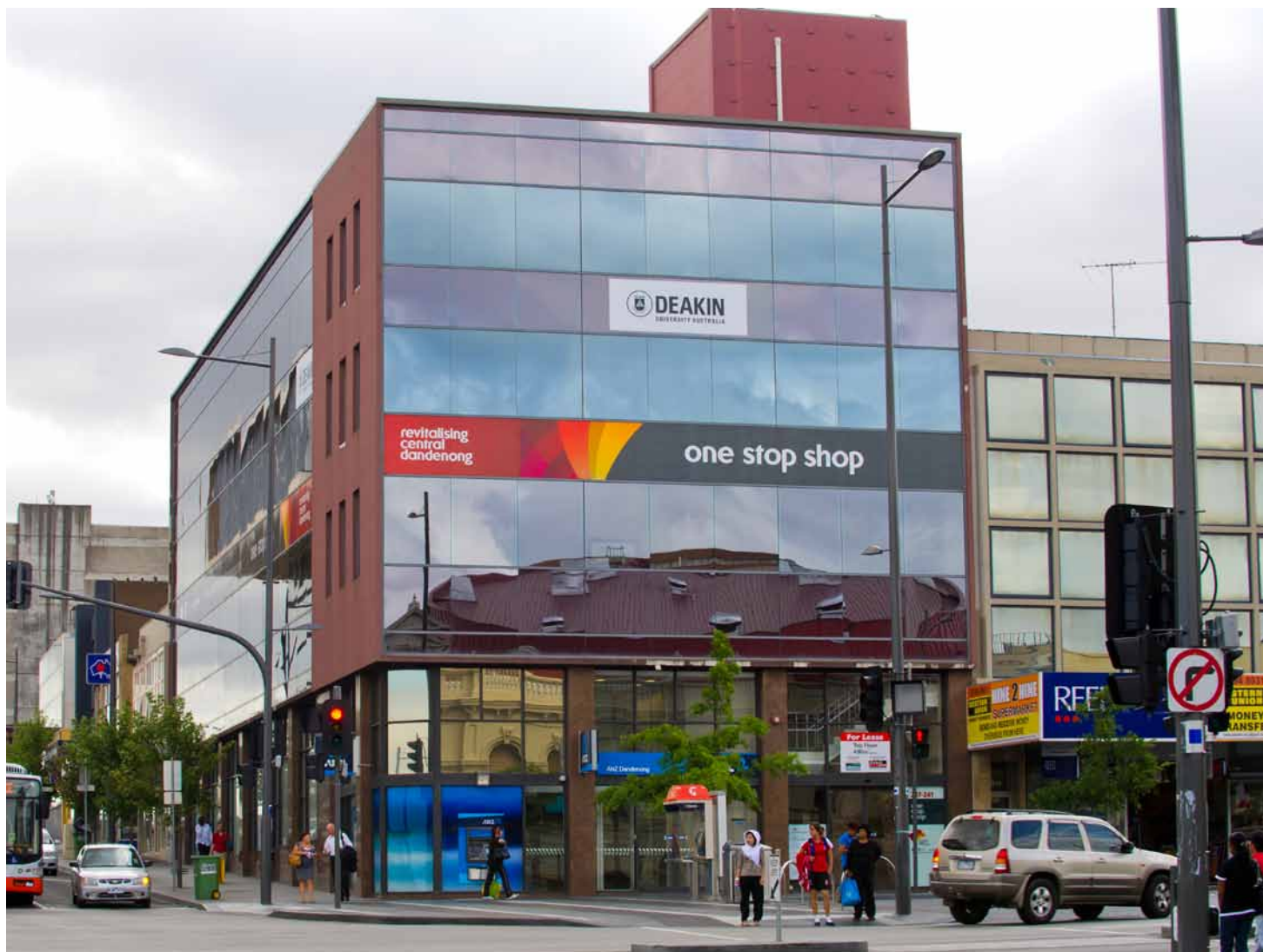
The recently opened Deakin Learning Hub, Dandenong
