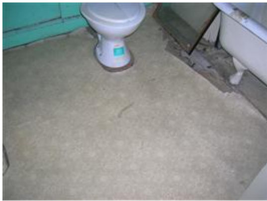
Photo No: Photo-05 Feature: Floor covering Material: Millboard Location: Western Beach Road; Building: 92-94; WESTERN BEACH RD - LEVEL 2; Room: BR.19 Sample Reference: 69311-8 Item Status: Positive
