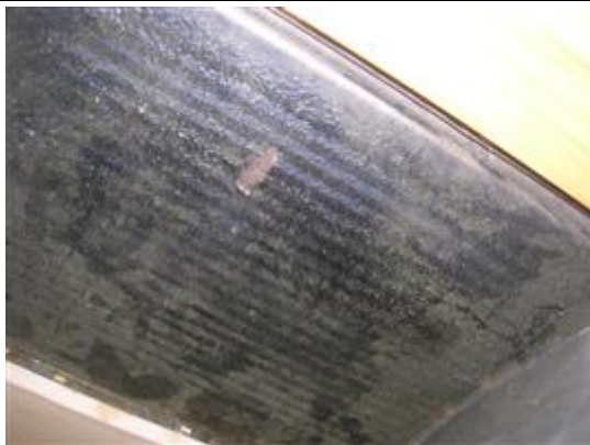
Photo No: Photo-10 Feature: Waterproof membrane Material: Bituminous membrane Location: Western Beach Road; Building: DCP; LEVEL 2; Room: C2.023 Sample Reference: 69311-5 Item Status: Positive
