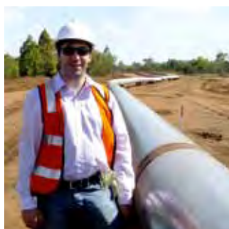
PhD student, Mr Facundo Varela is testing a new corrosion sensor in the field.
